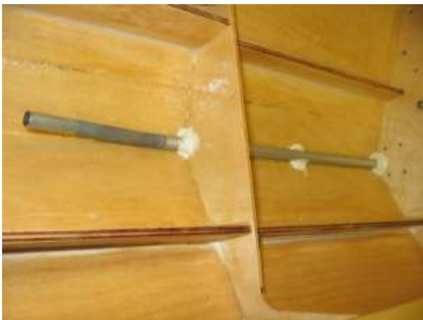
Notice the discolored area where the tube was heated.
