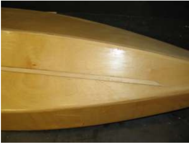
Front of strake. Keep parallel to keel.
