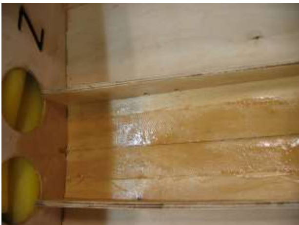
Seam glassed with 6 ounce cloth and epoxy resin.
