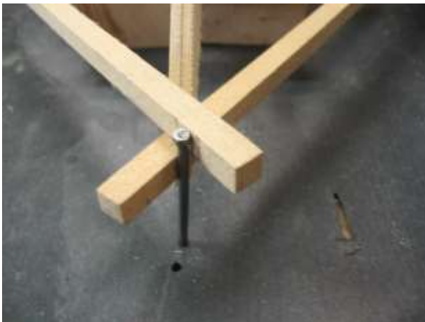
Nail to hold stringers.
